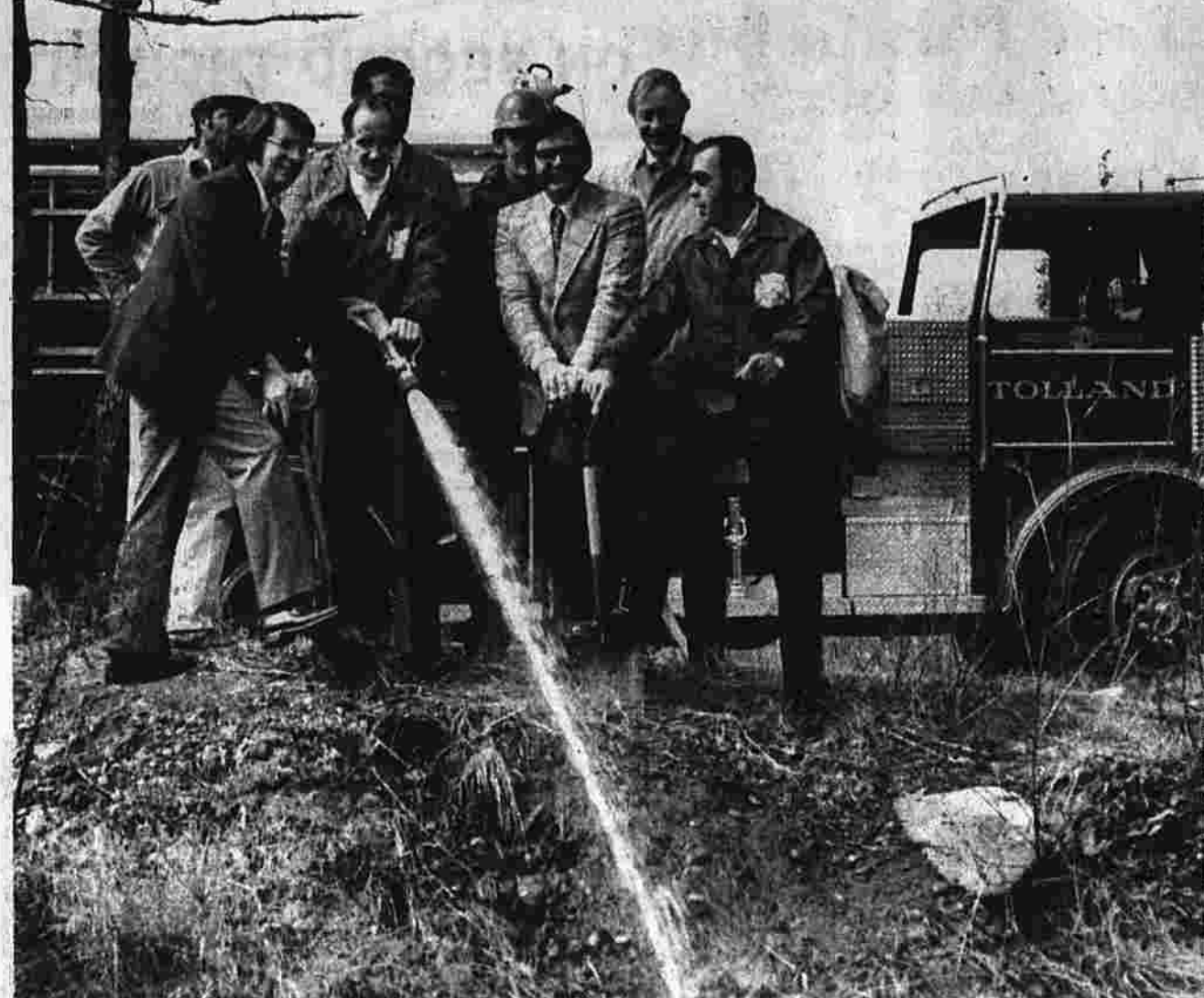
Participants of the recent groundbreaking for the $107,000 fire station off Gehring Rd. are: Selectman Kevin Cavagnah; building committee chairman Robert Clough; Town Manager John Harkins; and Fire Chief Ronald Littell. Shown in the back are Roger Gallher, architect; William Jamison, superintendent of the job; and Alphonse Patrick, general contractor of Building Innovations, Inc. (Photo by Lentocha)
